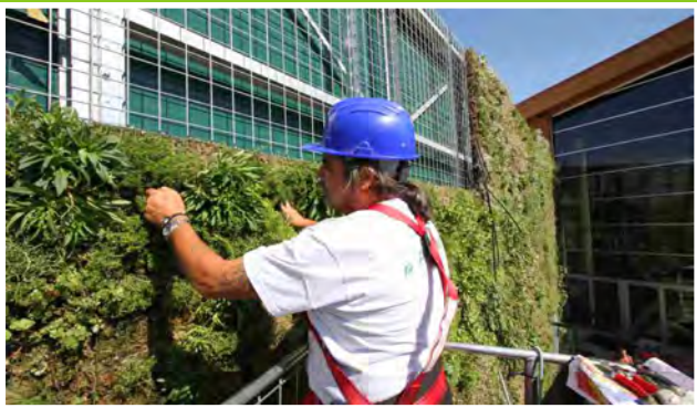
Posa in opera
